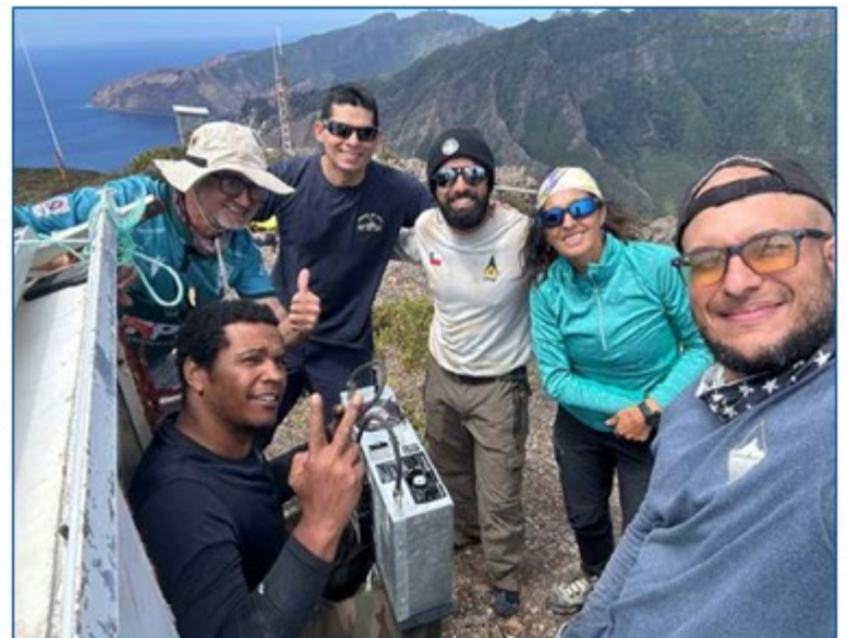
The team was able to repair the CONAF repeater on top of Cerro Alto: Cerro Centinela looms tall in the background.
