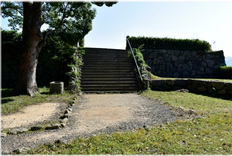
Tenshudai (keep foundation) The foundation was made, but the Tenshu was never built, as mentioned above.
