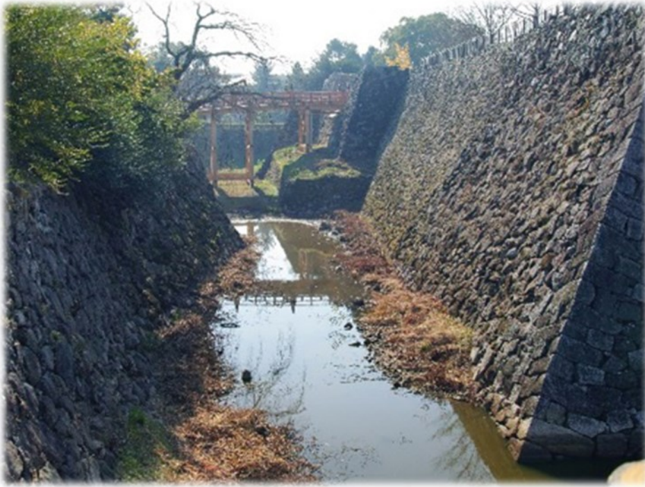
A view of the Gokuraku bridge and the inner moat.
