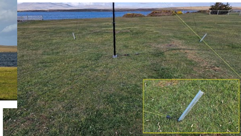
Figure 6 - 32 radials, 3.5 meters long and extra-large guy anchors.
